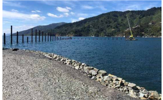
Piling progressing along the eastern breakwater.
