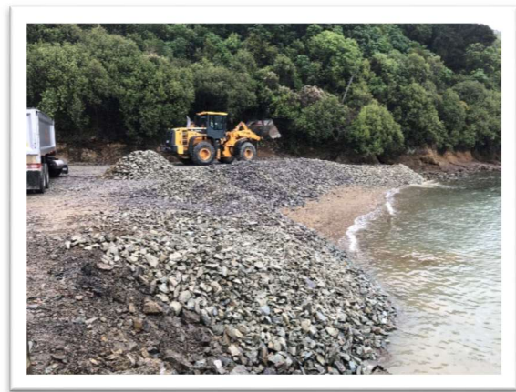
Photo 4 – First loads of material placed on site.
