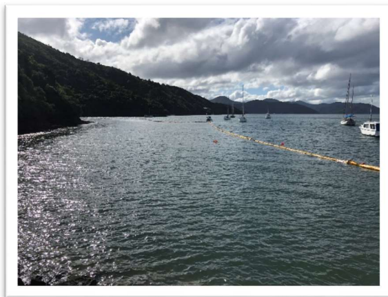
Photo 3 – Silt curtain re-installed following lockdown.
