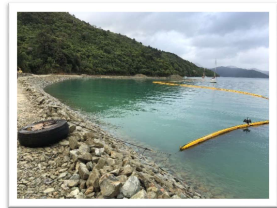
Photo 8 – Rock rubble placed to Ch.375
