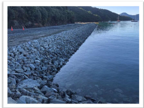
Photo 7 – Completed bund with armour rock
